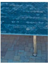
**LANDFILL LINER SHINGLES** were created through an experimental process, resulting in over 6,000 upcycled roof shingles, transforming unused local landfill liner into an essential resource. The project put to use an unwanted material and local labor.
